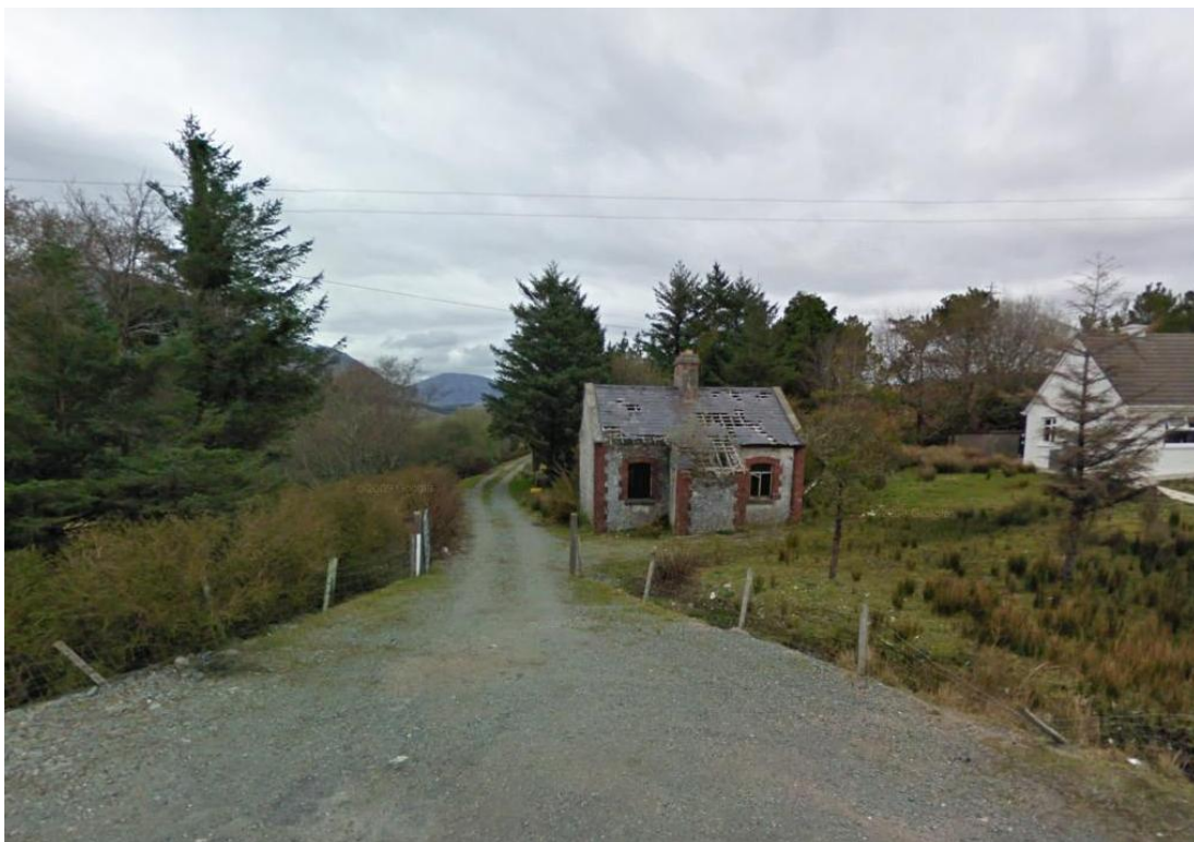
Image 14.10 Looking North East at Ch. 17+400
