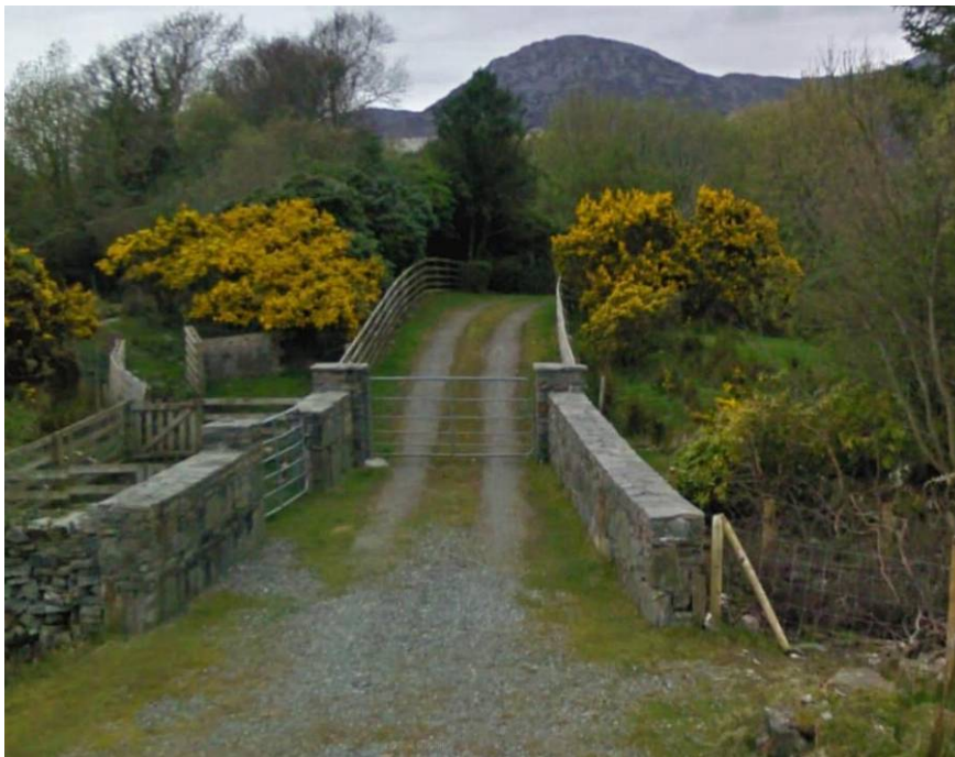
Image 14.7 Looking West at Ch. 14+800
