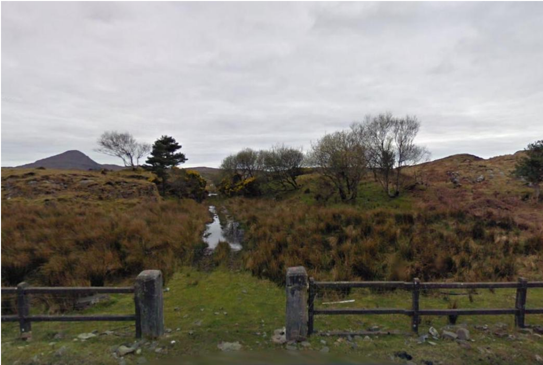
Image 14.11 Looking South West at Ch. 17+400
