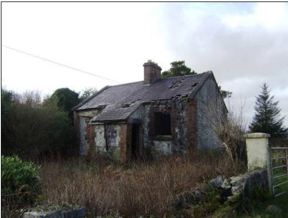
Image 13.5 BH 75, level crossing cottage (Ch. 34+500 to Ch. 35+450), facing south-west
