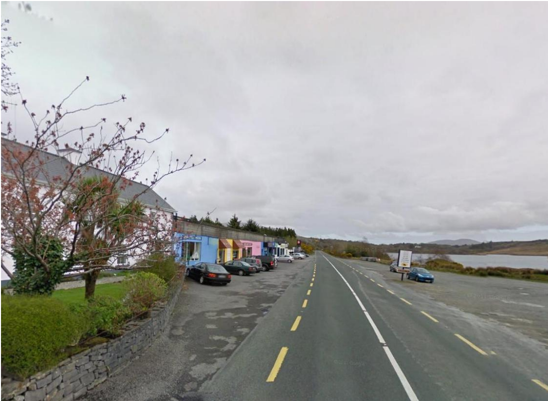
Image 14.13 Looking East at Ch. 21+200
