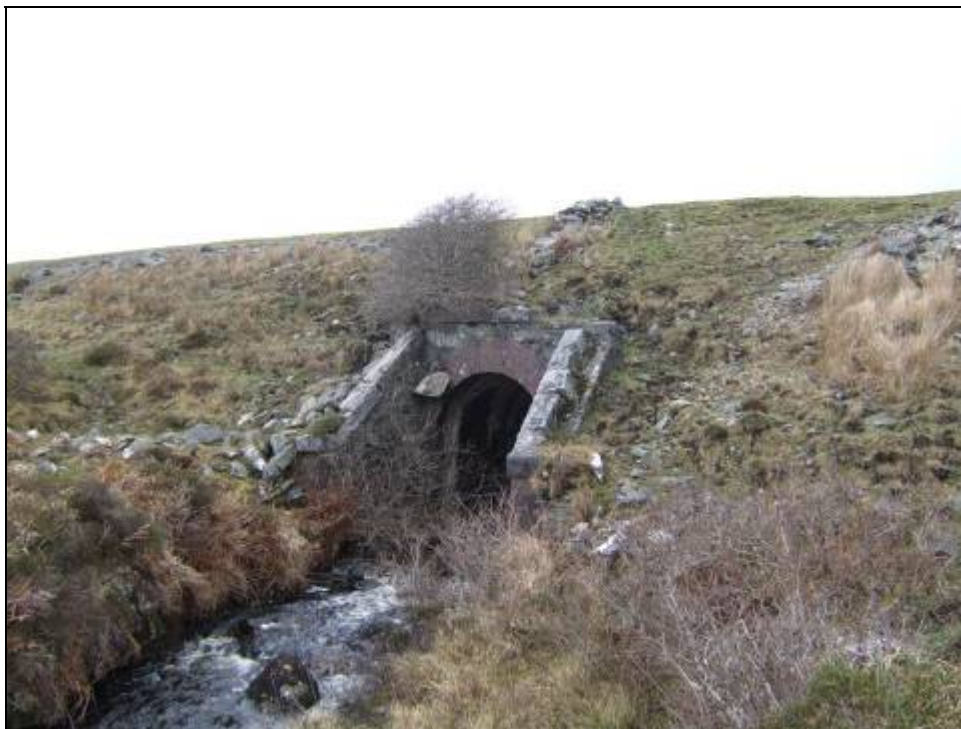
Image 13.3 BH 17, large culvert (Ch. 4+300 to Ch. 11+150), facing north
