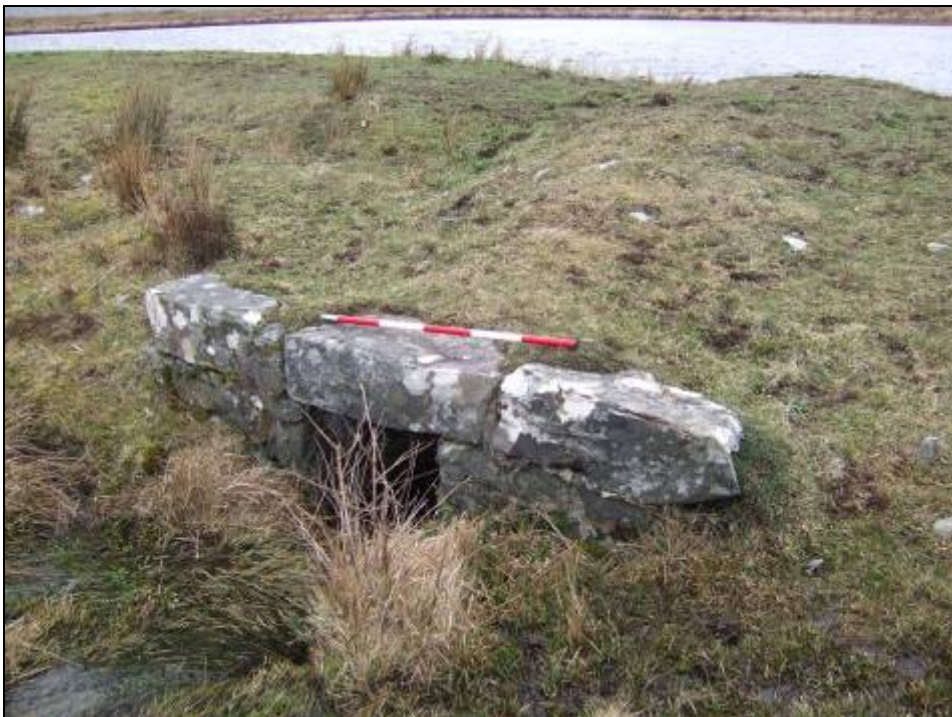
Image 13.2 BH 16, stone culvert (Ch. 4+300 to Ch. 11+150), facing north
