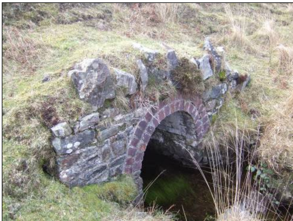
Image 13.4 BH 33, culvert (Ch. 15+150 to Ch. 17+400), facing south-east
