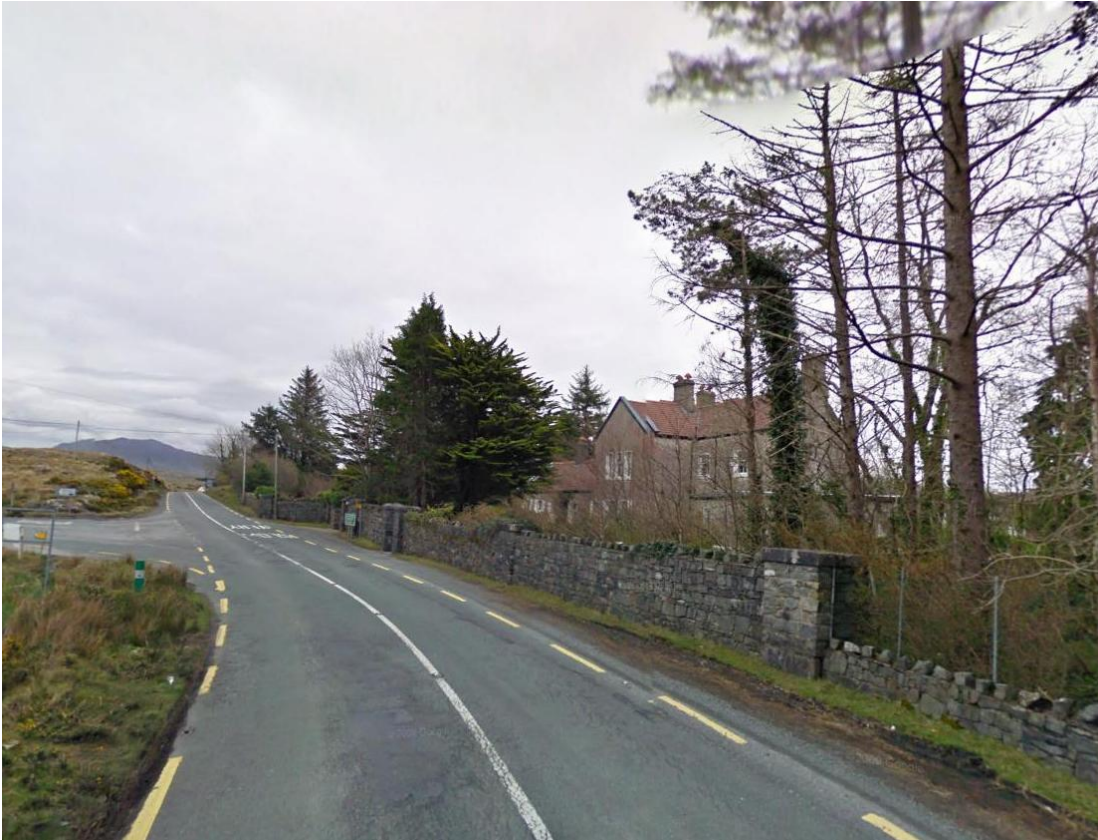
Image 14.12 Looking East at Ch. 20+200
