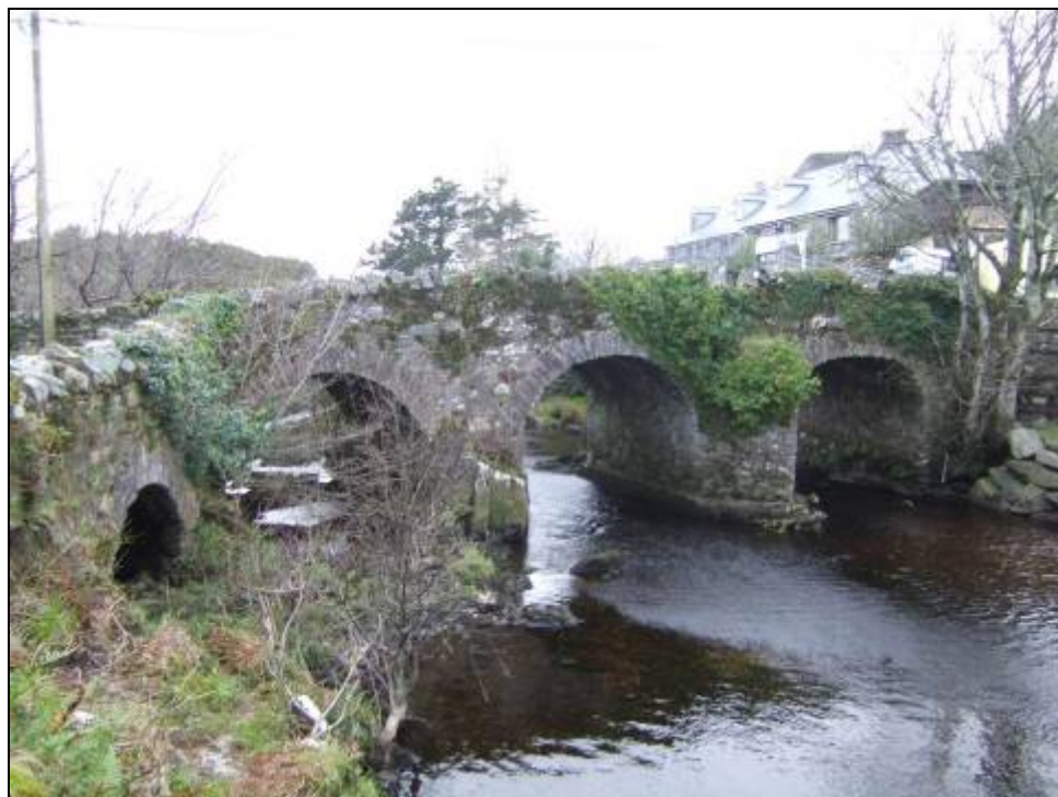
Image 13.1 BH 2, Ardbear Old Bridge (Ch 0 to Ch. 3+200), facing west
