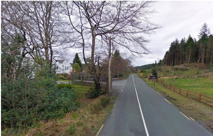
Image 14.6 Looking East at Ch. 12+600
