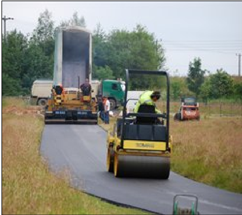
Image 6.2 Example of a similar final surface being laid
