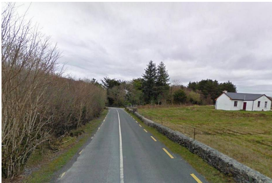
Image 14.8 Looking East at Ch. 15+000
