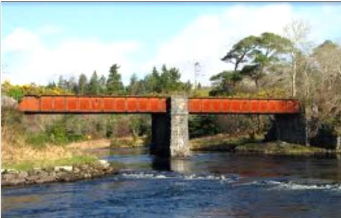
Image 6.7 Cloonbeg River Bridge currently in place
